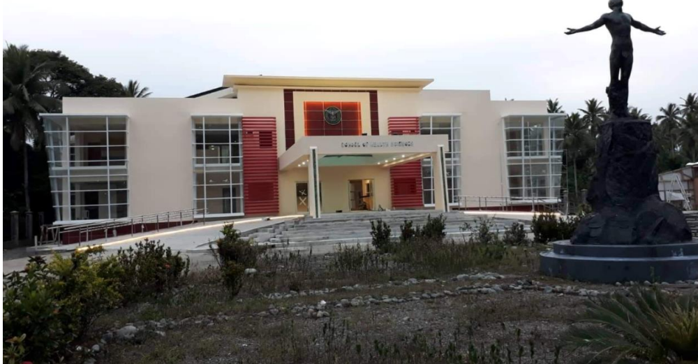
Figure 55 Existing Administration Building of SHS Baler
